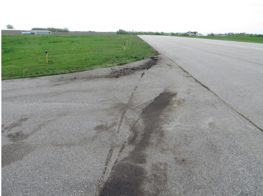
12Y CTA 001 (Oil Spill)
